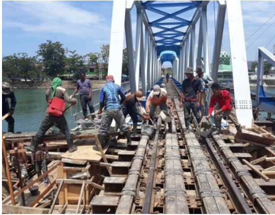
Gambar 6. Pengecoran wing wall
