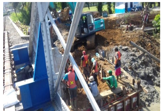
Gambar 4. Pekerjaan casing bore pile
