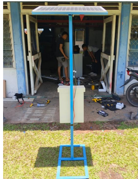
Figure 3. Implementation of power sources and support poles
