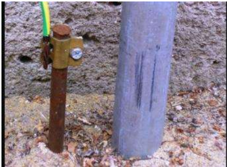
Gambar 1. Contoh grounding terpasang
