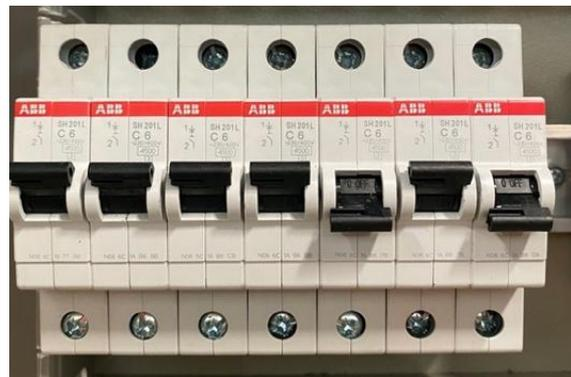
Gambar 3. Mini Circuit Breaker (MCB)
