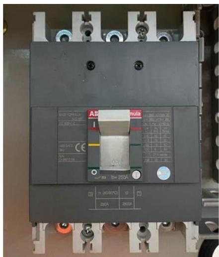
Gambar 2. Moulded Case Circuit Breaker (MCCB)
